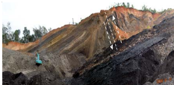
Figure 1. Structure condition in the investigated area
