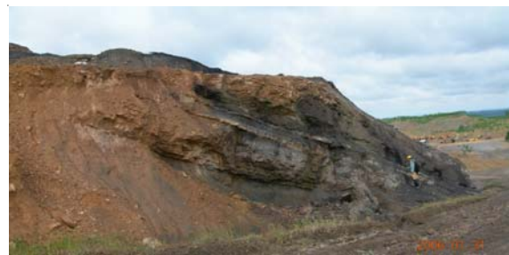
Figure 2. Location of geotechnical investigation at the low-wall
