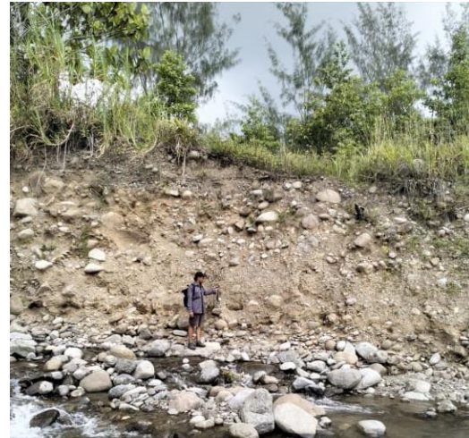
Figure 2. Slope to be repaired.
