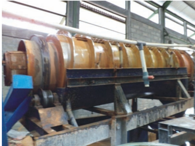
Figure 3. Photo of rotary drum scrubber (RDS)
